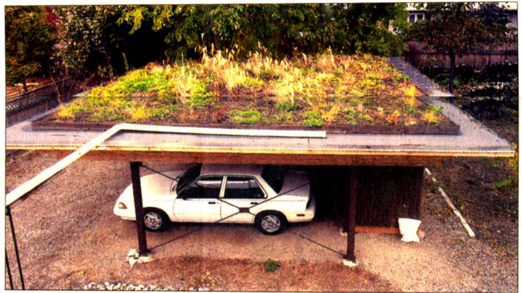
A carport and garden shed was built with an attractive "green roof" of hardy Canadian rye grass. A downspout from the home's roof diverts water to this garden.
